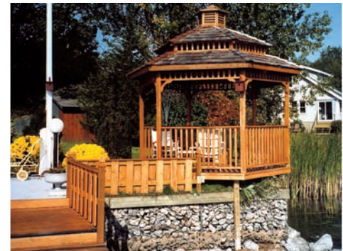
Capitalizing on the support of a stone breakwater, this 10' hexagon gazebo with optional 2-tier roof and cupola, built by Gene Manion of Mallorytown, Ontario, perches comfortably virtually on top the surrounding water
