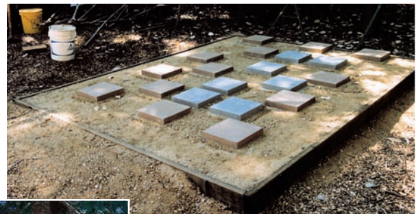
Here is a simple solution for uneven ground! 6' x 6' gardener foundation, built by Jerry and Judy Phillips of Bonny Doon, California
